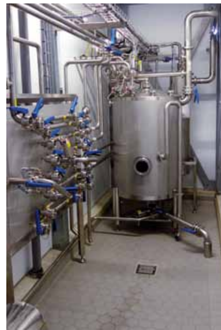
Fig. 3 A newly developed foam capturing system for up to eight tanks and a semi-automatic CIP distribution panel with swing pipes
