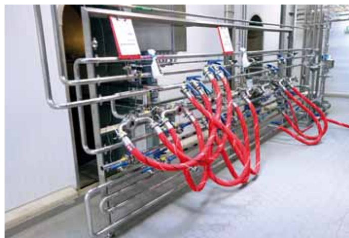
Fig. 4 Pipe manifold with hose connections and a position feedback control system for maximum flexibility and process reliability
