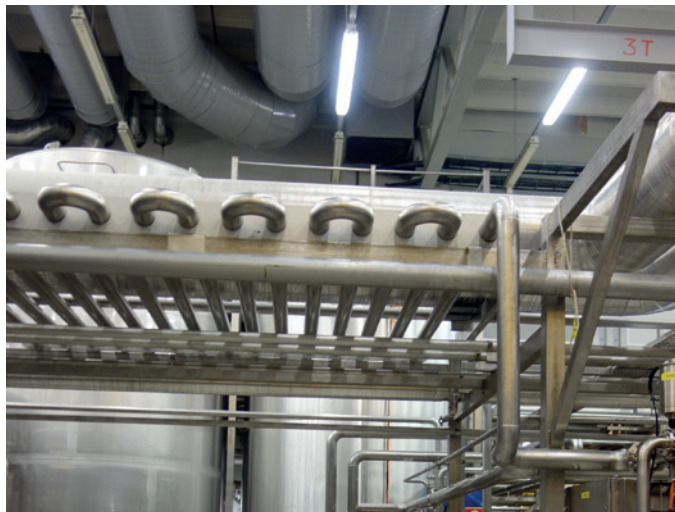
Fig. 3: Mixing section after bypass at the top of the picture; LoopulEX® Norway
