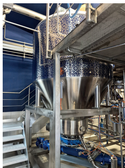
Figure 2: 40 hL mash-lauter tun with cone (left); Fürst Carl Castle Brewery, Ellingen Germany; view into the mash-lauter tun, special agitator with flow breakers and lauter sieve (right)
